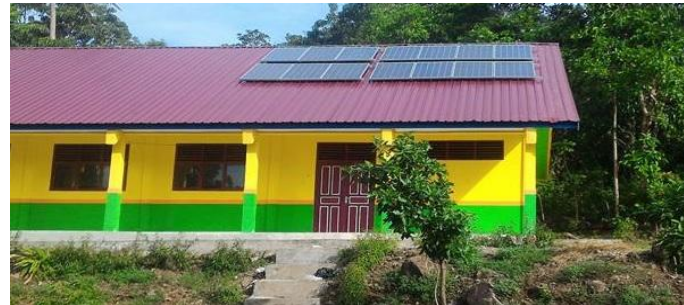
3.5 kWp PV with Hybrid inverter in Sulawesi
