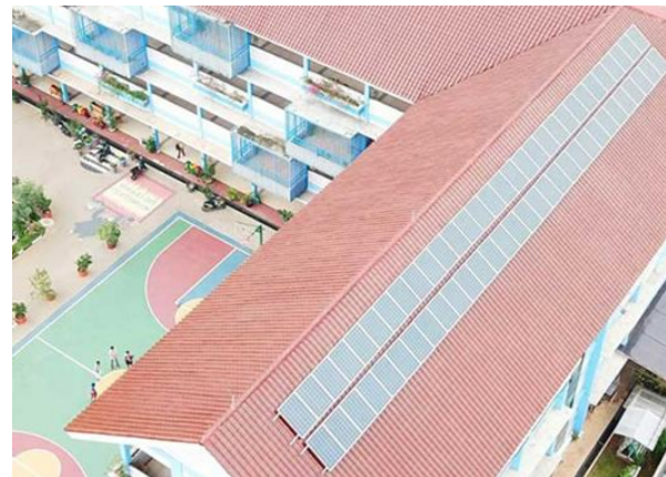
3.5 kWp PV with Hybrid inverter in Sulawesi
