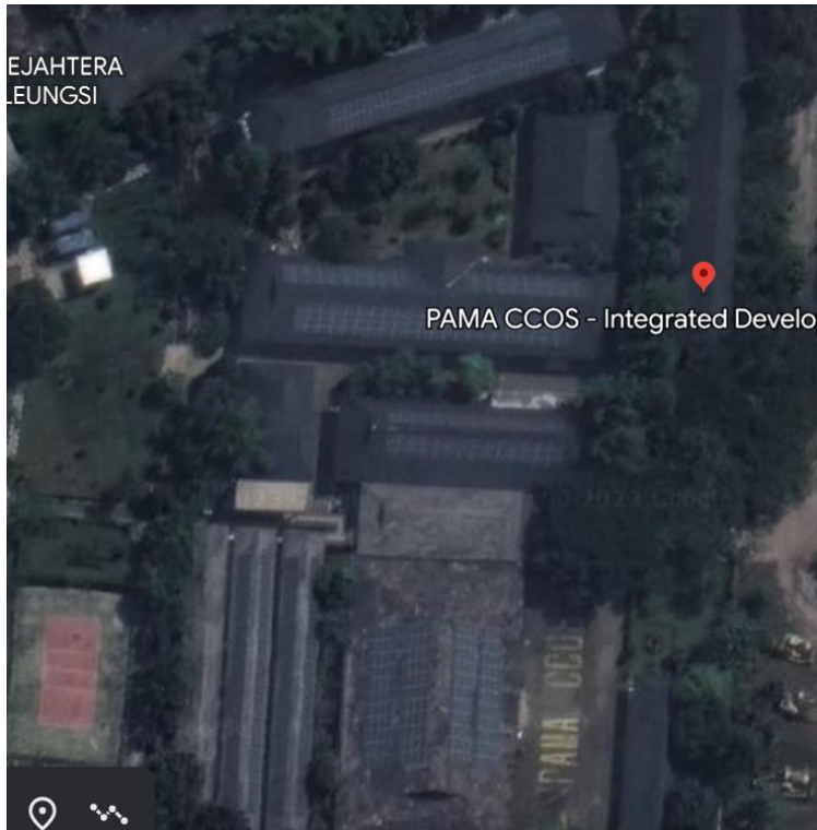
400 kWp PV Rooftop on PAMA Persada
